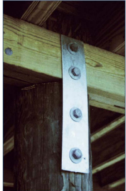
Metals corrode at a much faster rate near the ocean. Always use well-protected hardware, such as this connector with thick galvanizing.
