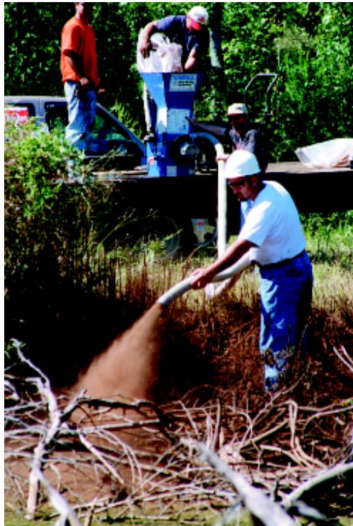
Spraying milled bagasse on an oil spill may become a standard practice for remediating oil-contaminated wetlands.
